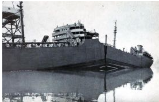
Figure 1: Crack failure of WWII Liberty Ships.
